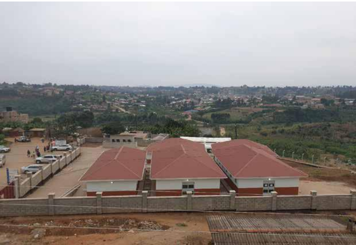
Picture showing the aerial view of the site. Photo credits: Barigye Celestine
