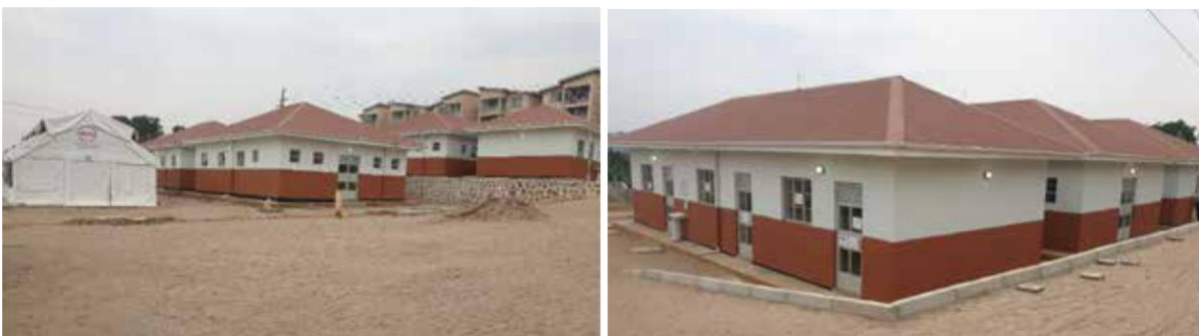
Progress of works on the COVID-19 Treatment Unit. Photo credits: Barigye Celestine
